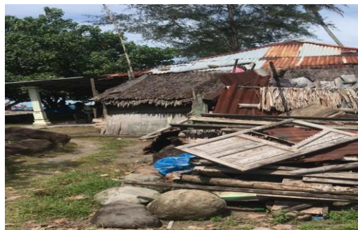
Fig. 1 Condition of community settlements affected by abrasion on Naras beach
