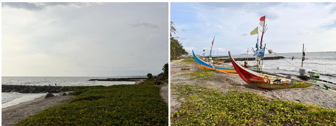
Fig. 4 Grip stones as wave barriers that have been installed on Naras Beach
