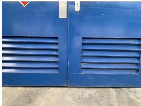
Figure 2. Air ventilation at the bottom of the door
